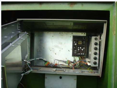
Fit New Door, Connect Looms and Fit Aerial ...
