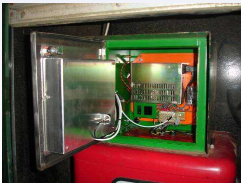
Fit New Door, Connect Looms and Fit Aerial ...
